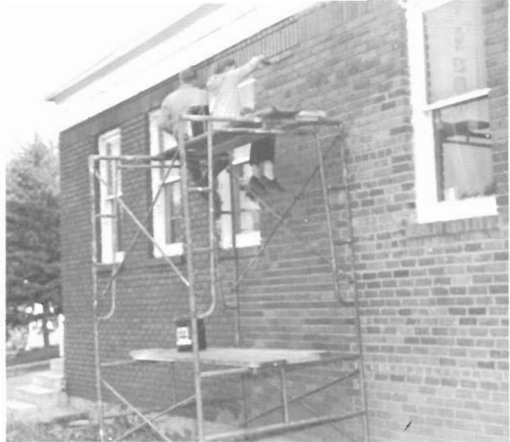
The maintenance building receives a coat of paint from Larry Christensen and Ted Toms.
