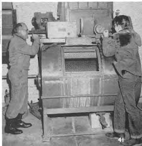
Keith Hagen pours coal into the stoker as Kenny Pierson shovels it into the furnace to keep our buildings warm.
